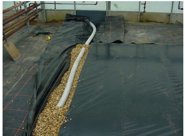
Photos 5 - 8 Preparation of demonstration scale capillary flow bed
