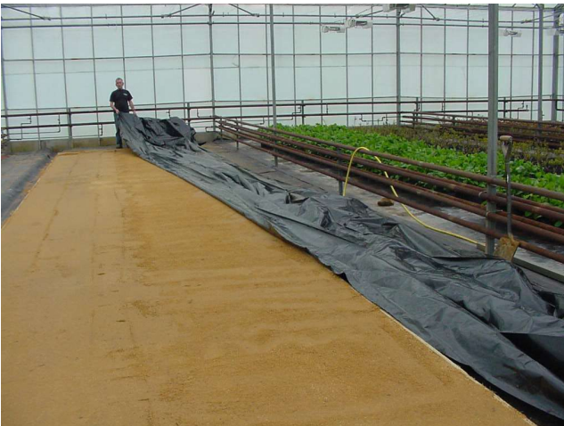
Photos 5 - 8 Preparation of demonstration scale capillary flow bed
